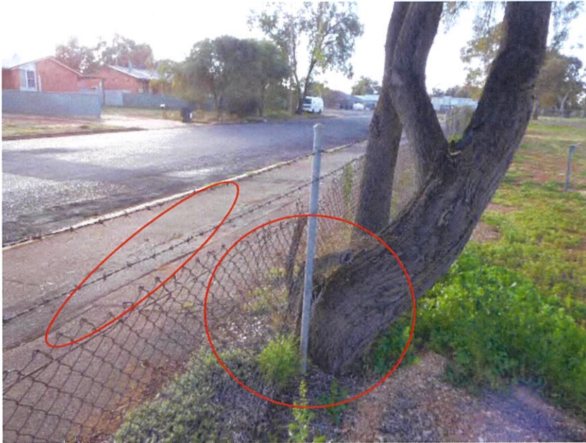
Photo 8 – Lower stem system of Tree 9 - Acacia salicina (Cooba). IF the fence is to be removed then do not pull post out of the ground – cut it off and retain it. Removal this close to the tree may destabilise the tree particularly if there is a concrete footing on the post. Also noting that some root systems were likely cut on the footpath recently for some trenching activity.
